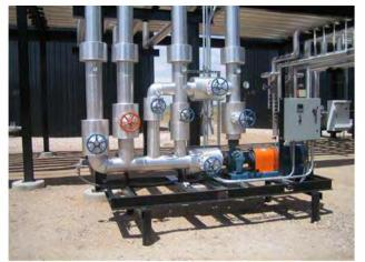
ECF designed and engineered the warm oil loop system to assist in maintaining product temperatures by recirculating thermal oil through a closed loop method.
